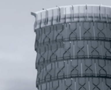
Detail of the fixing and reinforcement system of the plates.
